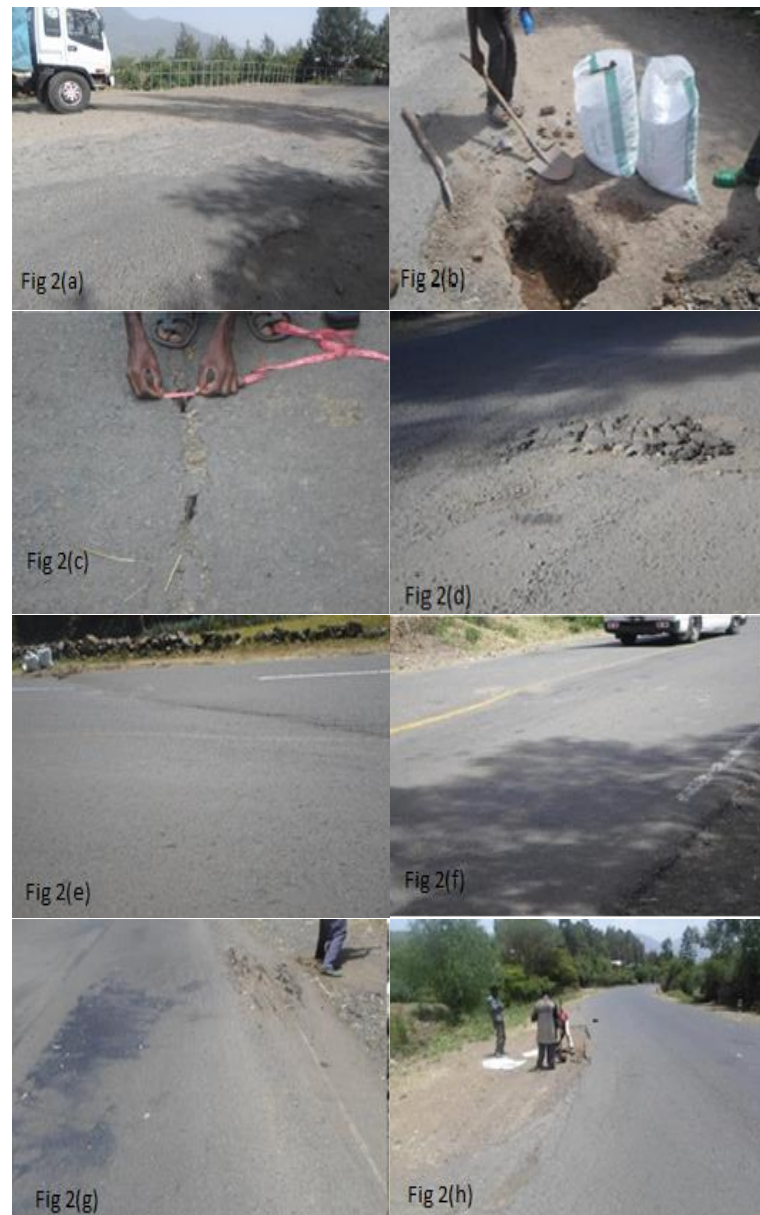
Fig. 2(a): Photograph image showing pavement distress of a road segment between Kemissie and Dessie; Fig.2(b): Sample -I collection from pavement dislodgement; Fig.2(c): Sample-II collection from transverse crack; Fig. 2(d): Sample-III collection from patched pavement; Fig. 2(e): Sample-IV collection from non-uniform road surface; Fig. 2(f): Sample-V collection from distorted road surface; Fig. 2(g): Sample-VI collection from sheared road surface; Fig.2(h): Sample-VII collection from potholed pavement.
