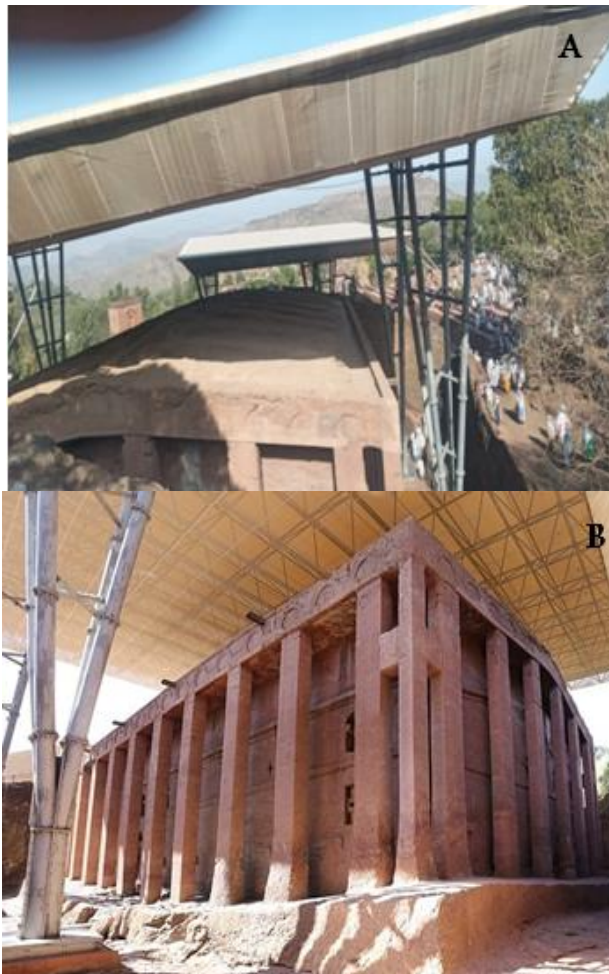
Figure 4: The Roof (a) and Installed Shelter (b) of Bete-Medhane-Alem – church -Source: Author December (2020)
