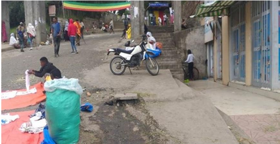
Fig. 11 The Manhole opened and release liquid waste at the main gate of St. Gebriel Church
